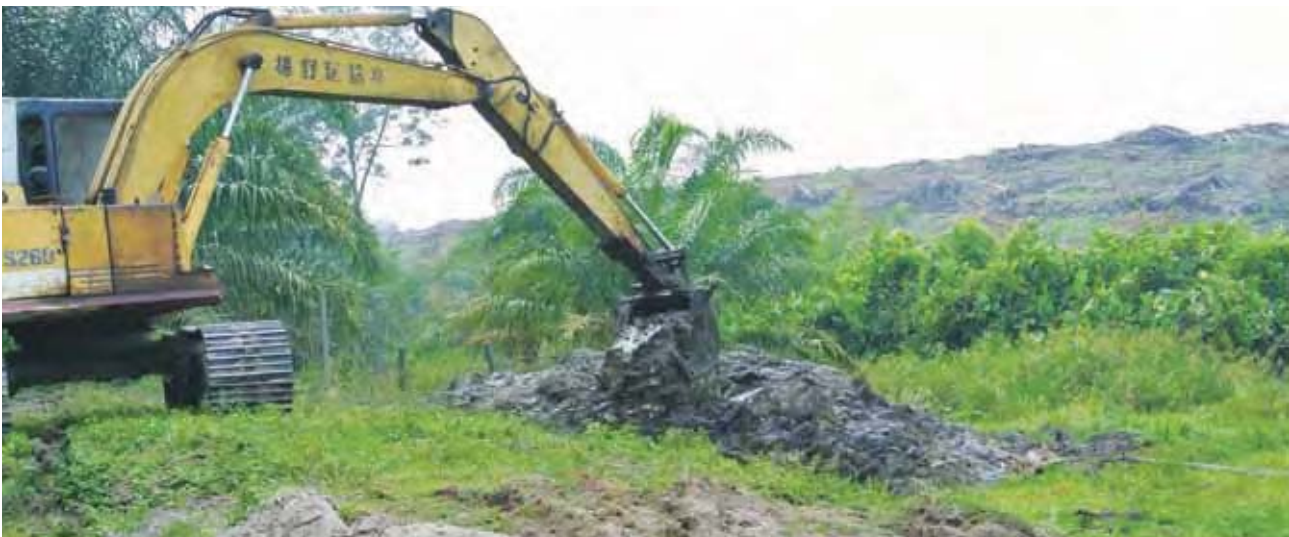
Security – Trenches being dug around the estate perimeter to strengthen security.
