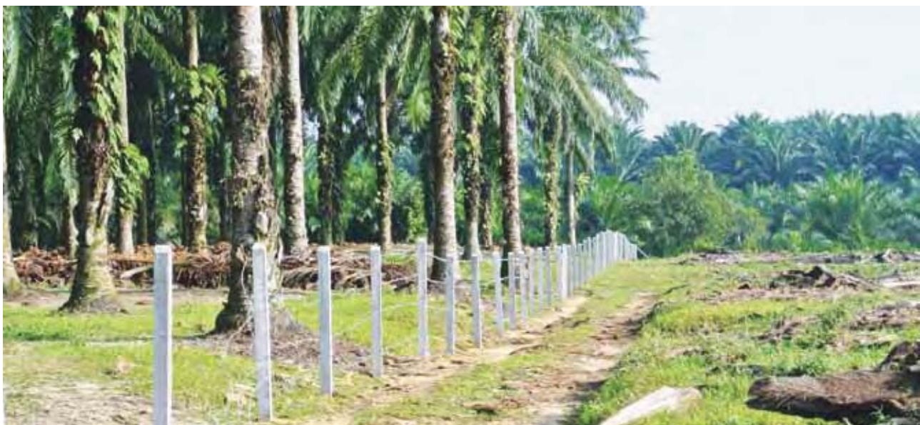
Security – Construction of barbed wired fences in progress
